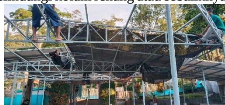
Gambar 5 proses instalasi atap
